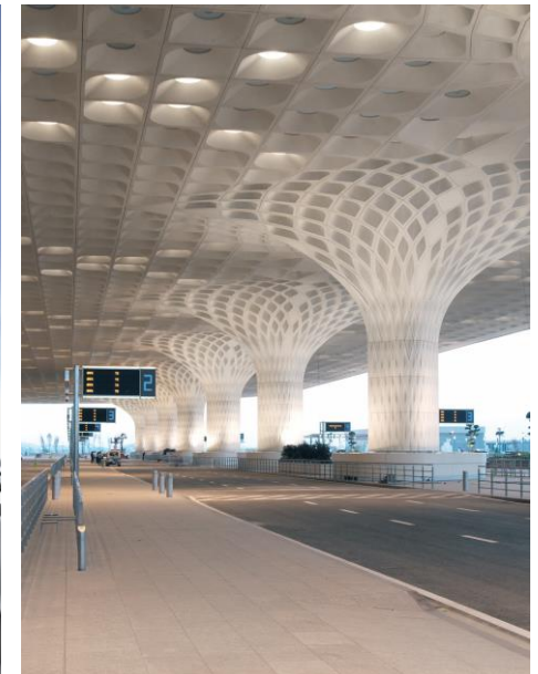
Chhatrapati Shivaji International Airport Terminal 2
