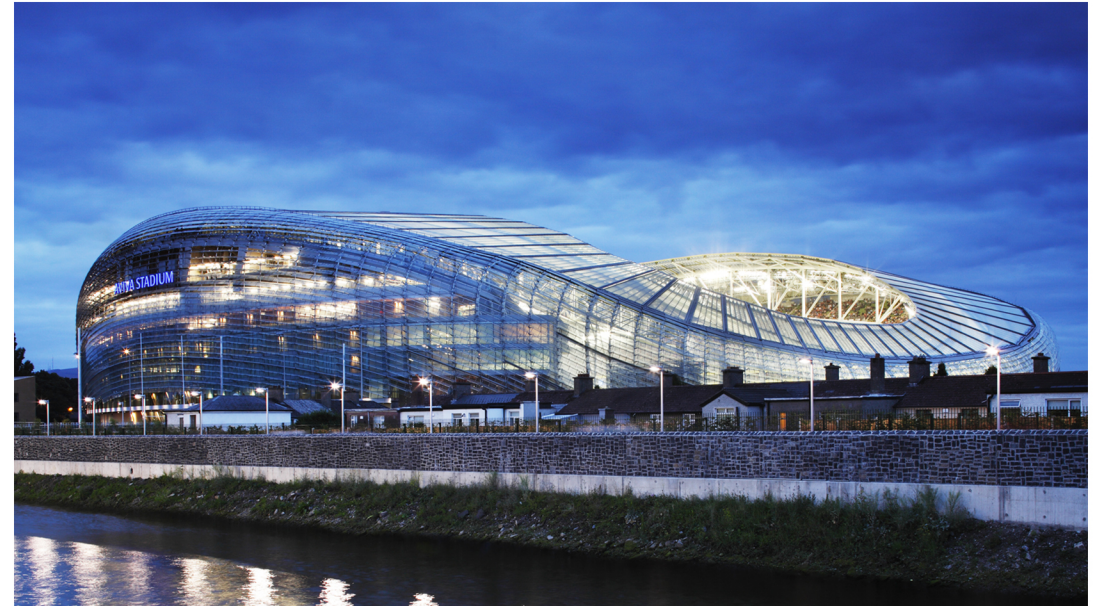
AVIVA STADIUM Architect: Populous & Scott Tallon Walker
