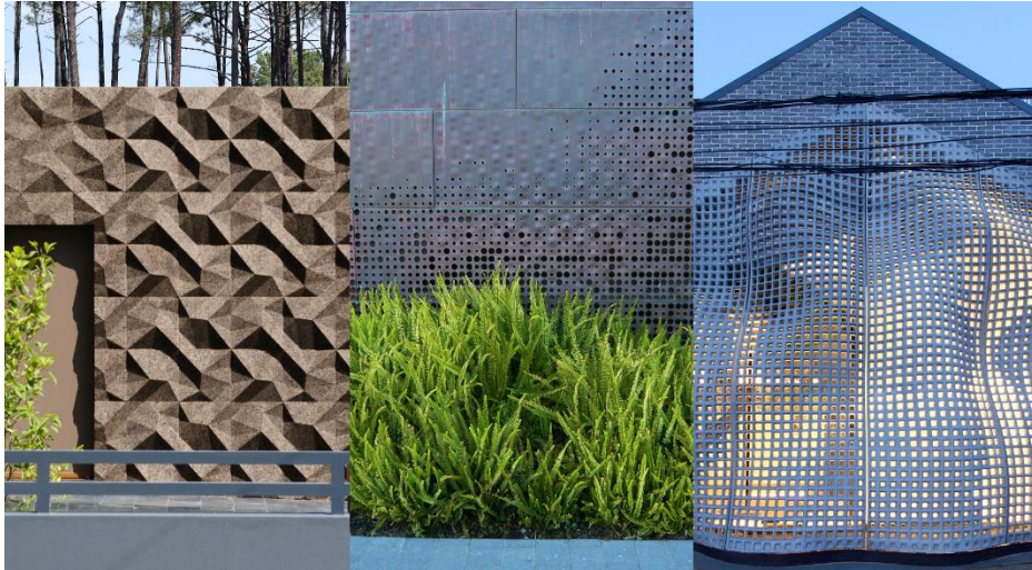
Fig. 3. Subtractive manufacturing: cork facade (©GenCork and Sofalca); De Young Museum (©David Basulto via flickr); MaoHaus facade (©XiaZhi ou ©Antistatics).
