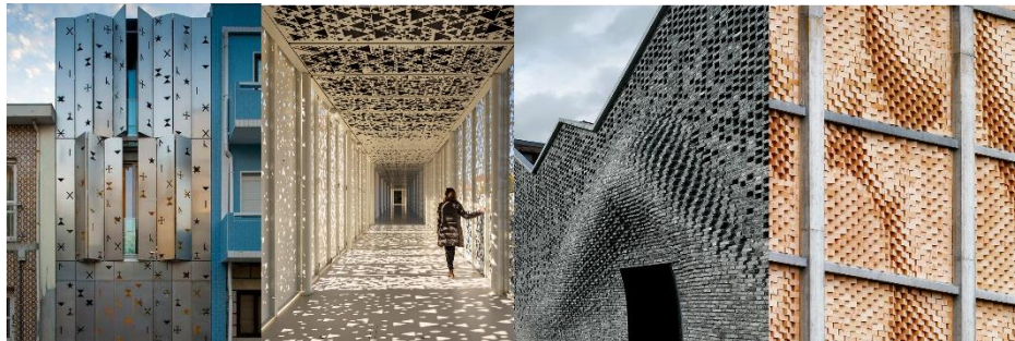
Fig. 5. Cutting and robotic manufacturing: House 77 by dIONISO LAB (©FG|SG Fotografia de Arquitetura); Megalithic Museum by CVDB Arquitetos (©Fernando Guerra | FG+SG); Chi She Gallery (©Su Shengliang ou ©Trevor Patt); Winery Gantenbein (©Christoph Kadel via flickr).
