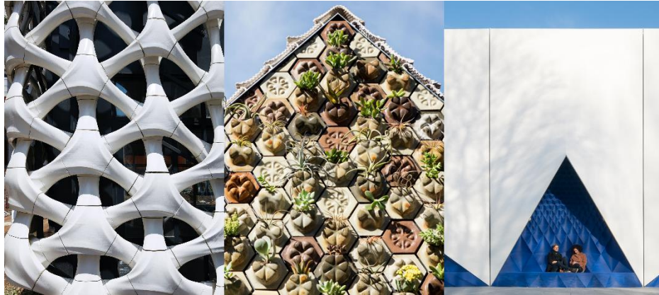
Fig. 2. Additive manufacturing: Arachne 3D printed facade (©Archi-Solution Workshop); House of 3D Printed Curiosities (©Matthew Millman Photography / Emerging Objects); EU Building 3D printed facade (©Ossip van Duivenbode).
