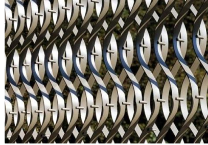
Fig. 13. Element's Distortion: Undulated Elements - Visitor Pavilion National Museum Palace in Het Loo, Apeldoorn, Netherlands.
