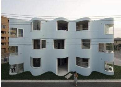
Fig. 4. Facade Geometry: Facade with horizontal waving - Apartment house in Tokyo.
