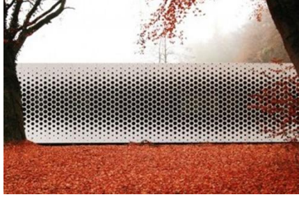
Fig. 2. Facade Geometry: Straight Facade - Formestelle Office Building, in Töging am Inn, Germany.
