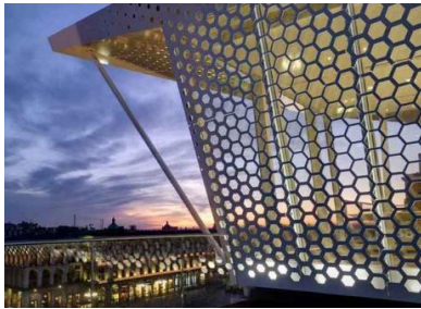
Fig. 9. Element's Geometry: Hexagonal Elements - The Cube, in Milan, Italy.
