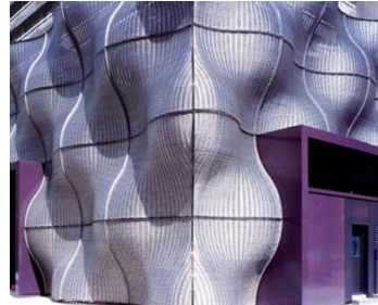
Fig. 5. Facade Geometry: Sinusoidal and cosinusoidal Facade - Boiler House at Guy's Hospital, in London, UK.
