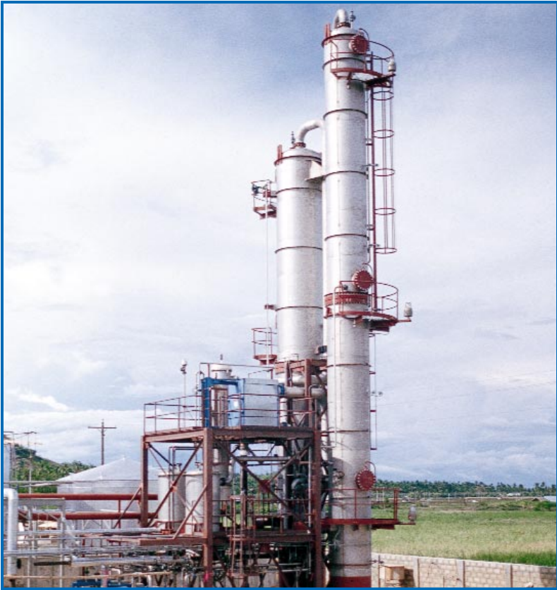
Figure 12. Two-effect isopropyl alcohol recovery system.
