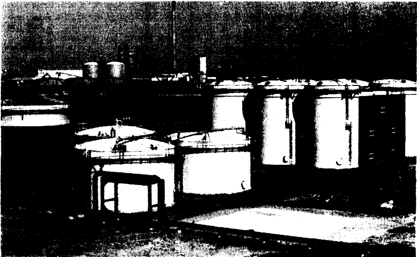
Figure 23.24. Aerial view of the Bayer Tower Biology® reactors (far right) at Bayer's Brunsbüttel works.
