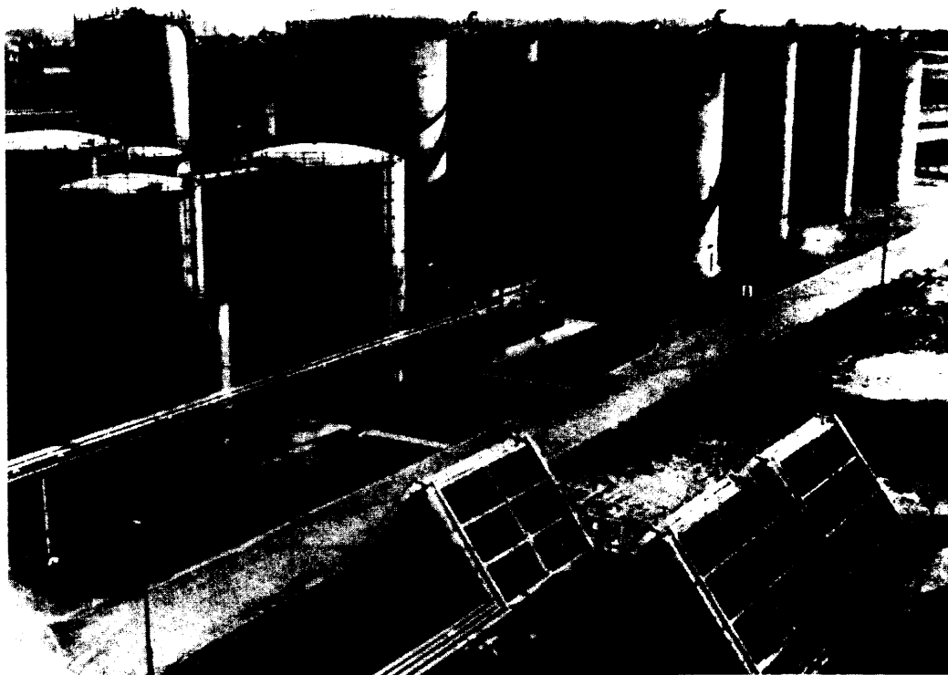
Figure 23.26. Bayer Tower Biology® facility at a refinery operating according to the principle illustrated in Fig. 23.25.
