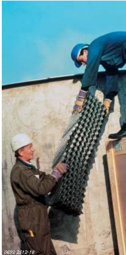
0692 2512-18 Revamping of a vacuum column with Mellapak
