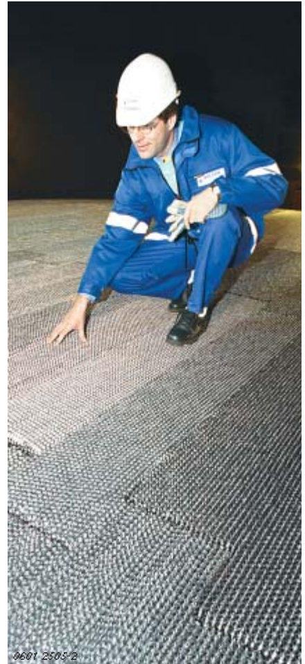
0601 2505-2 Inspecting packings after installation
