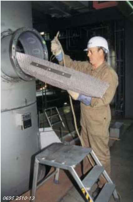
0695 2510-13 Installation of packing
