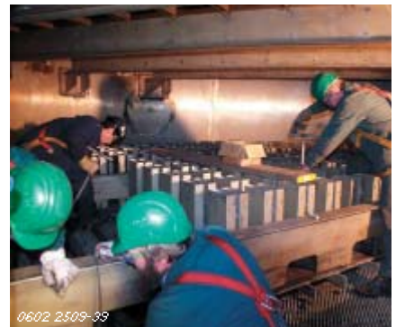
0602 2509-35 Installation of the liquid distributor
